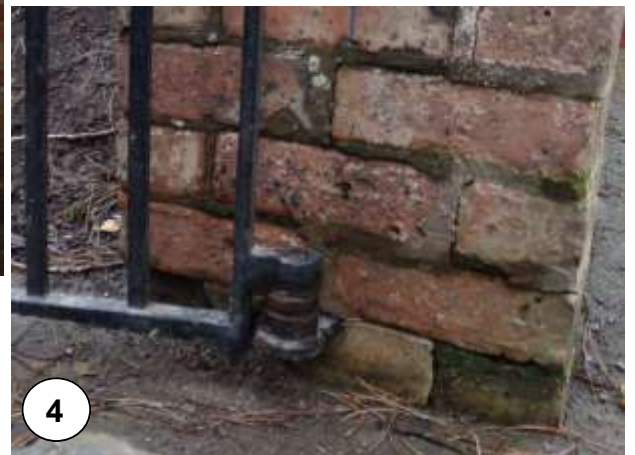
Figures 2-4. 2. Church gates. 3. Gate column patched with modern brick and showing stone cap and hinge bracket support. 4. Lower hinge bracket for western gate showing adjustment ring and decayed brickwork.
