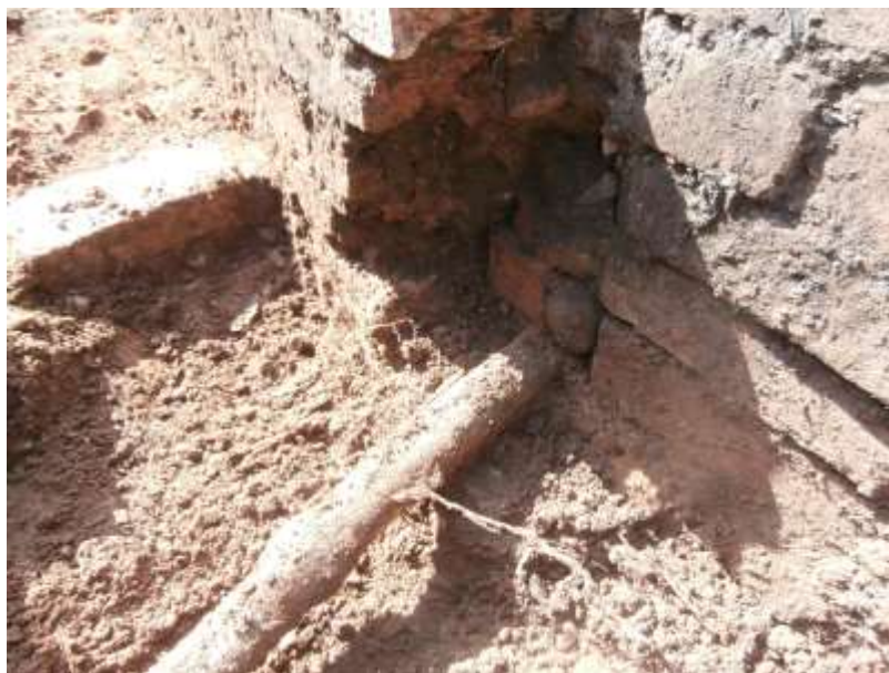
Figure 32. Trench 7. Outside eastern wall of cellar. Lead pipe with wiped joint where it passes through the cellar wall.
