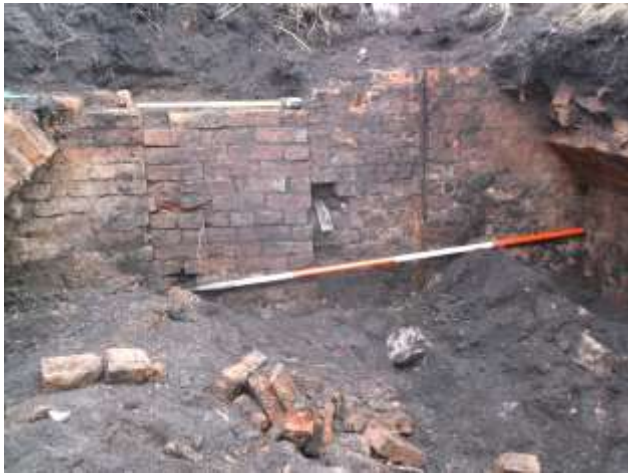
Figure 15. East wall of cellar. Note lead pipe and straight joint in brickwork.
