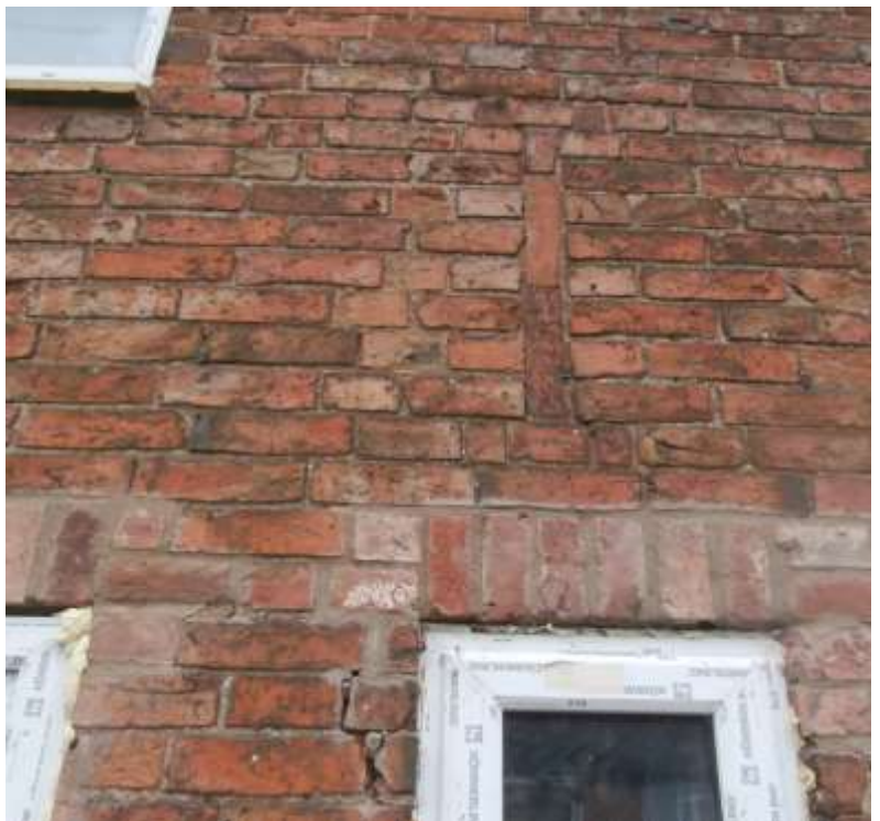
Figure 2. Bricked-up arrow slit ventilation hole.
