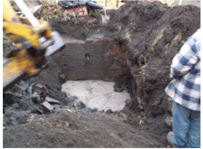
Figure 16. East wall of cellar. Note top of arch just above water level.
