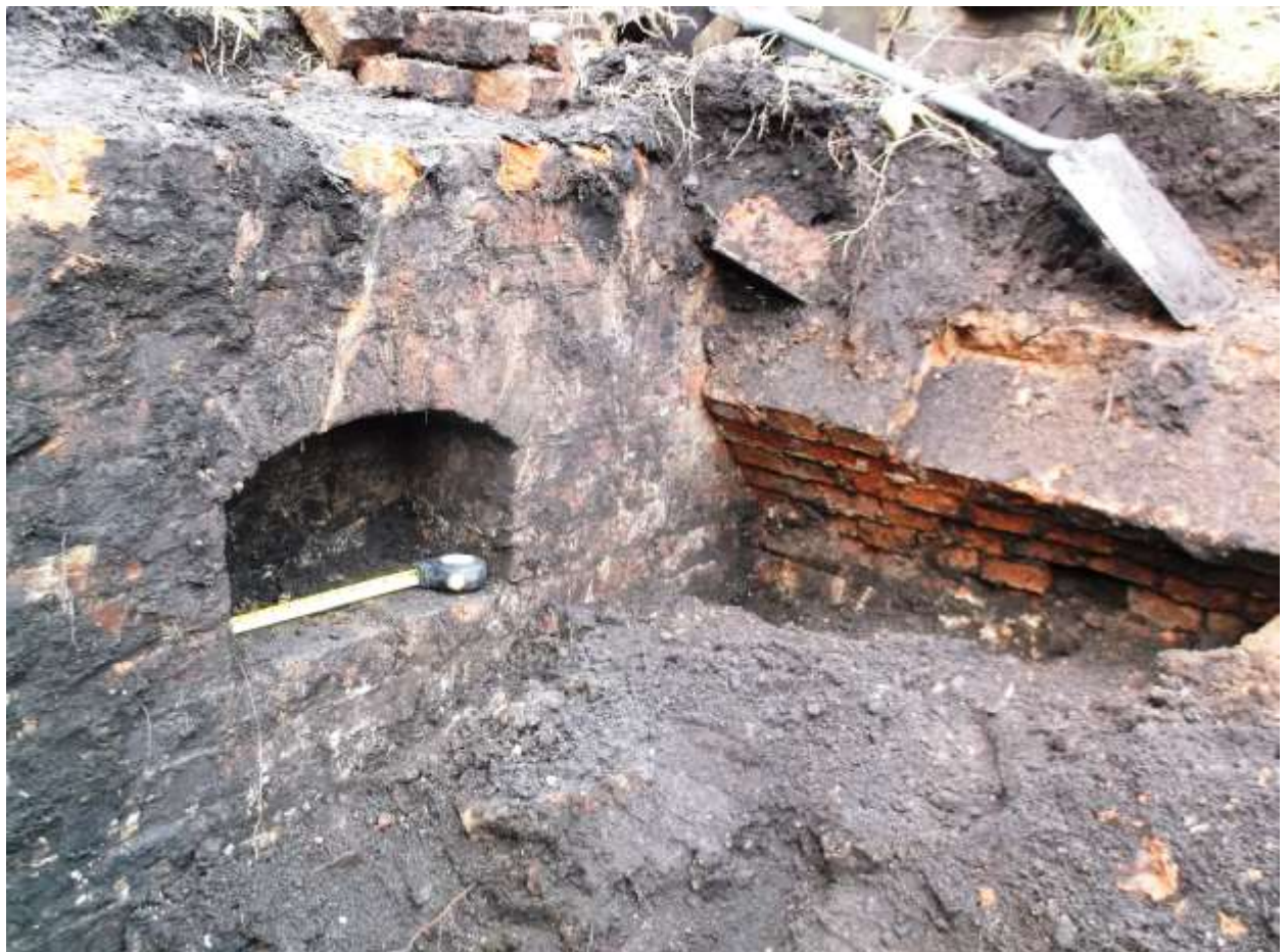
Figure 11. North-west corner of the cellar showing recess and bottom of collapsed arched roof.
