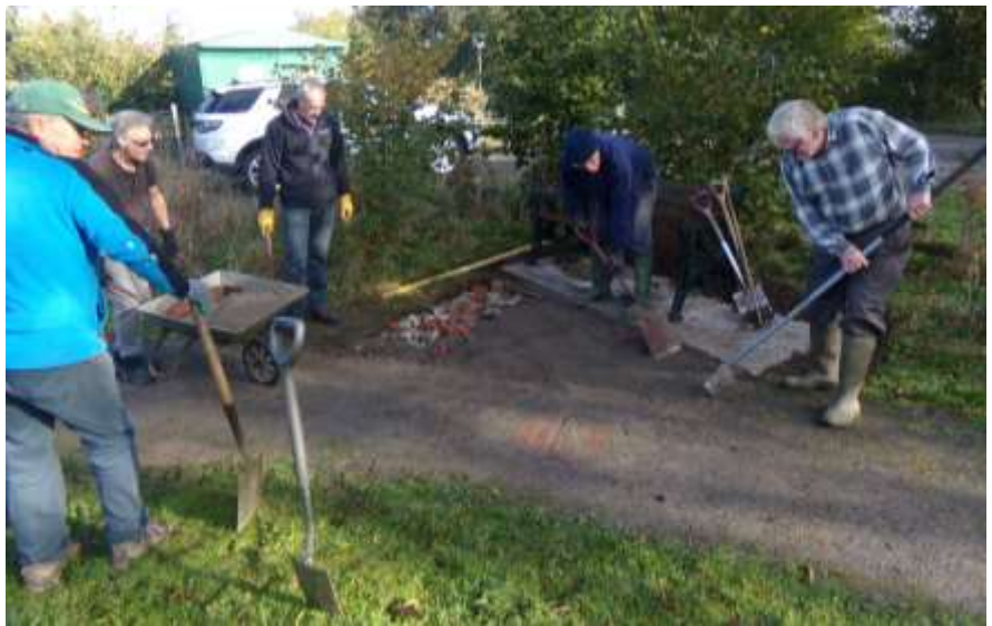
Installation of bench seat Carlton Diamond Jubilee Orchard 28th October 2019
