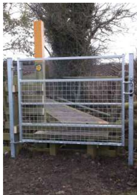
New hand gate on footpath S68
