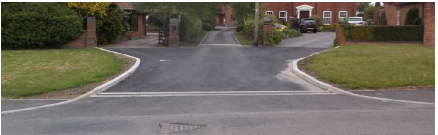
East Green kerbing works
